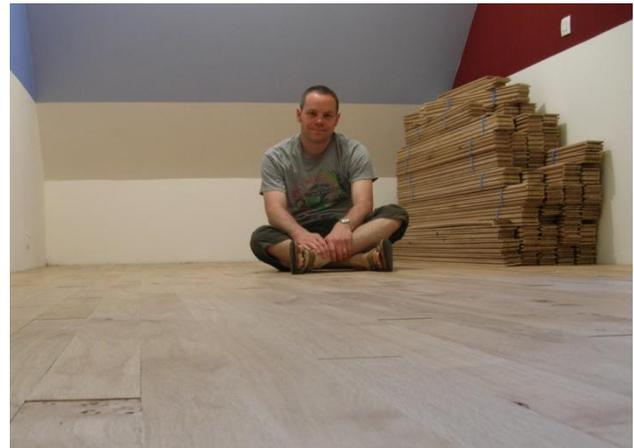
The floor has been leveled, insulated, and the hard woods are laid! All that remains is sanding and finishing the floor, then installing the wall molding. We'll all be happy when it's finally done!
